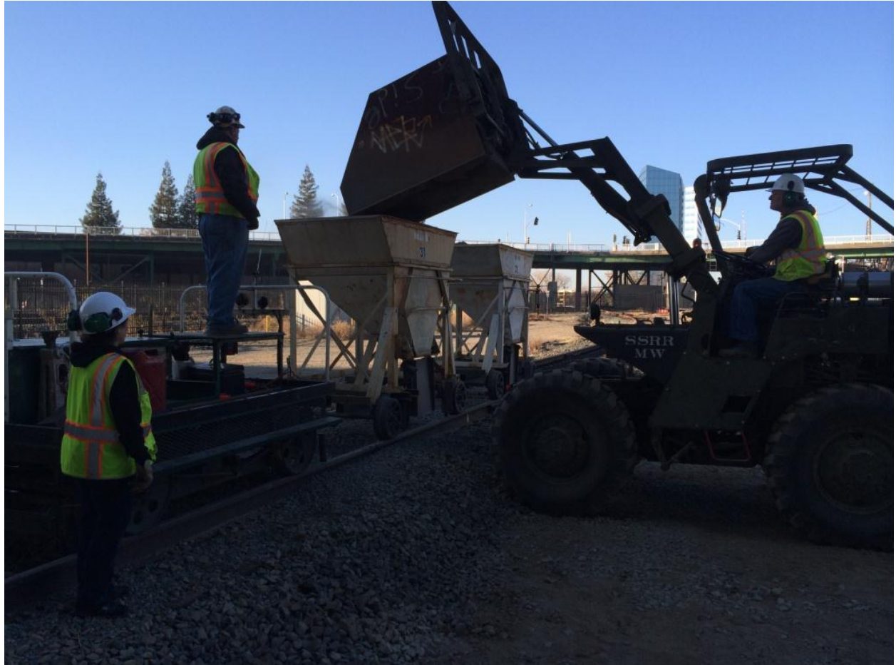
Pam and Mike F. monitor the filling of ballast hopper by Steve in the Green Machine
